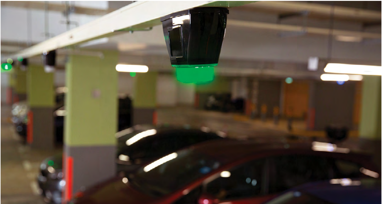
Lot availability is signalled by the overhead light indicators, enabling motorists to locate available lots quickly.
