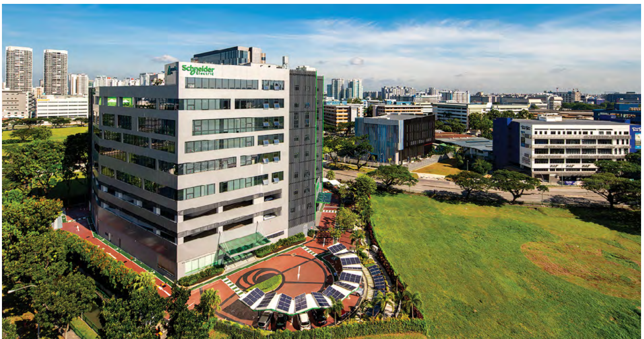
The Schneider Electric Building located in the Kallang industrial belt in Singapore has 5,000 connected Internet of Things points and is 100% solar powered during daytime. It is the regional headquarters of the company. Image: Schneider Electric.
